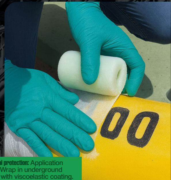
Complex geometry: 45° elbow repair on a tailings pipeline.
